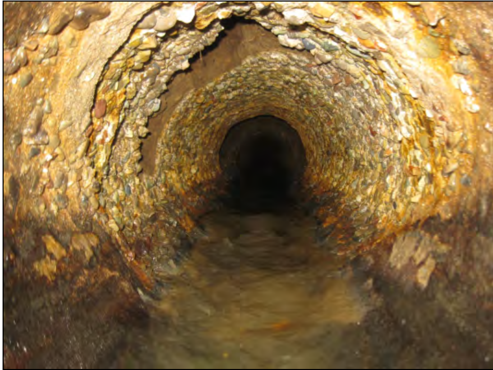
East Influent Pipe
