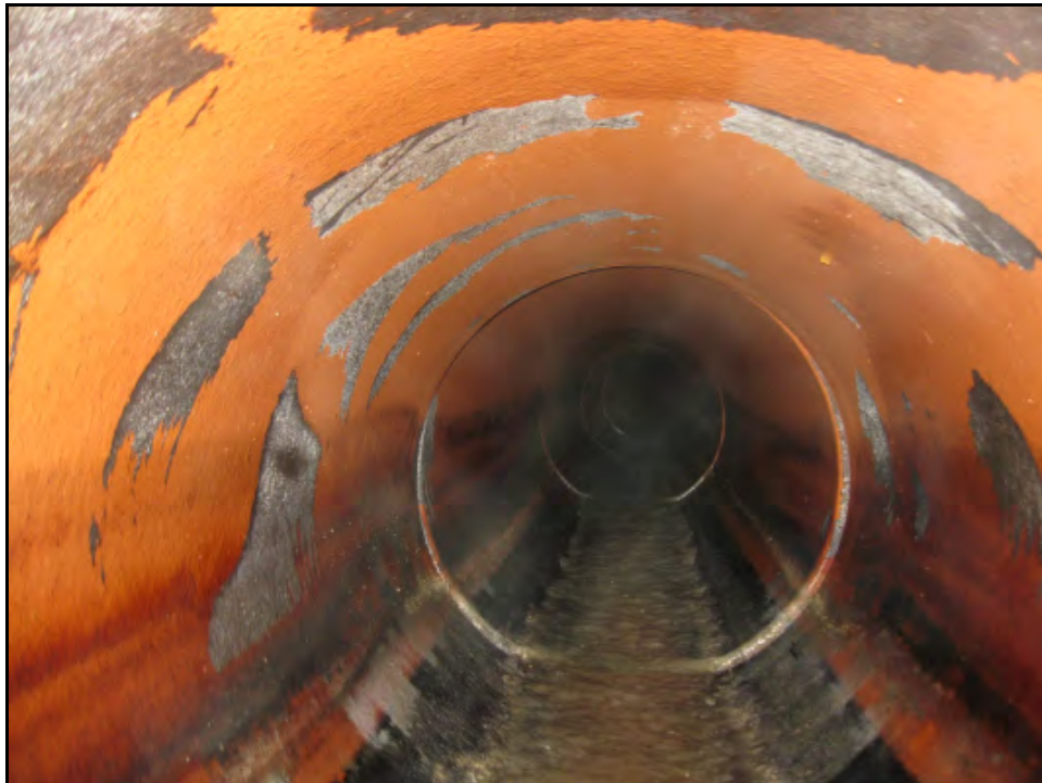
South Influent Pipe
