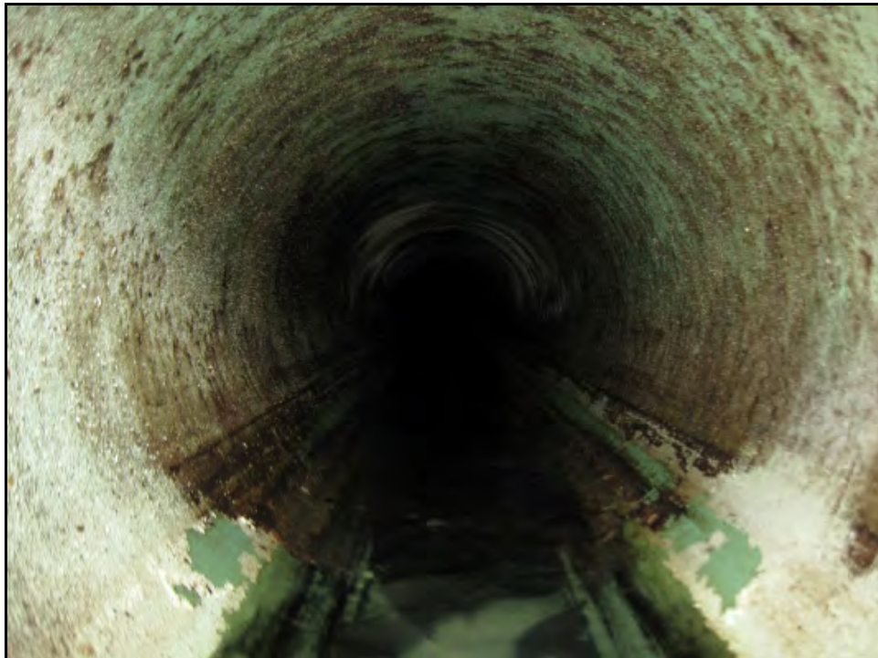
North Influent Pipe
