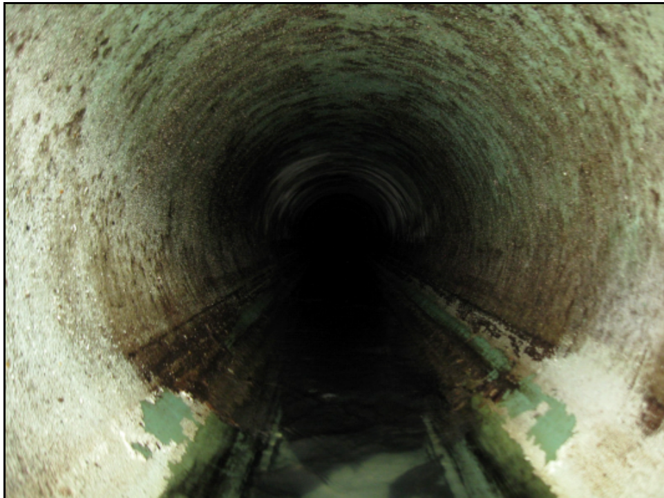
North Influent Pipe
