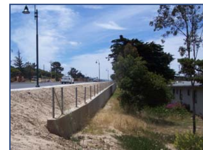
COMPLETED RETAINING WALL
