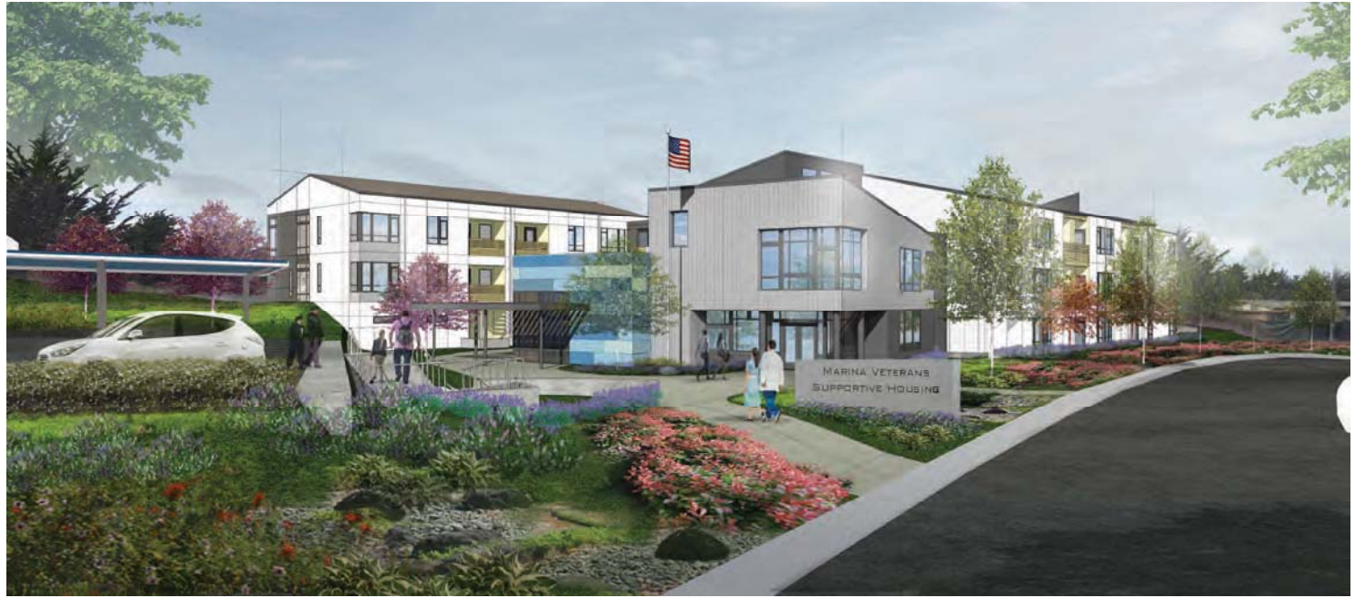
VIEW FACING NORTHWEST ALONG MILLER
