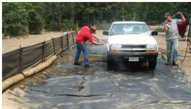
Contain waste water when washing vehicles to prevent spreading invasive plant parts.
