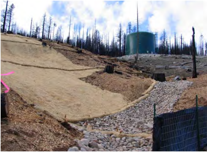
Erosion control with weed-free materials post-fire is important for reducing invasive plant spread.
