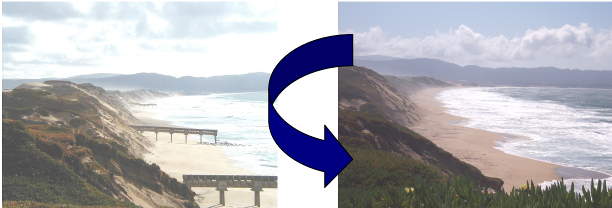
Storm drainage outfall removal — Before and After
