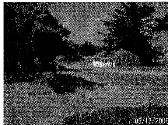
Building removal at the Imjin Office Park site
