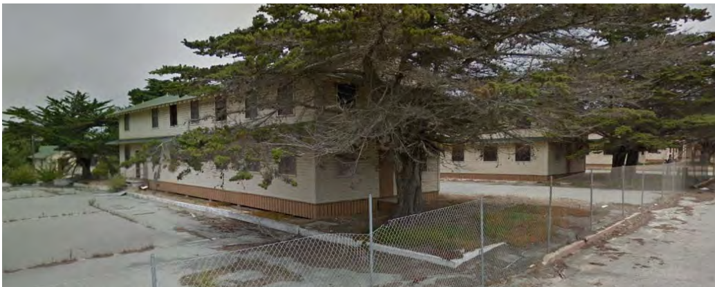
Abandoned barracks located adjacent to First Avenue
