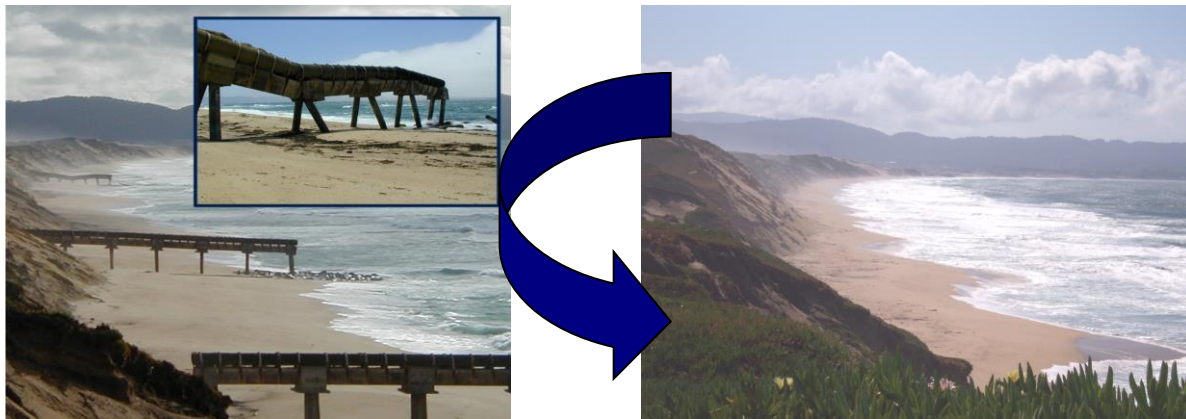
Storm drainage outfall removal – Before and After
