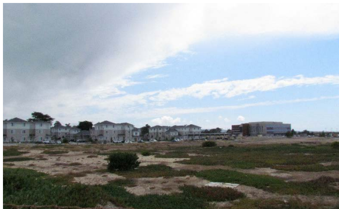
Building Removal by FORA opened land for the Dunes on Monterey Bay housing and new Veterans Hospital on 8 th Avenue.
