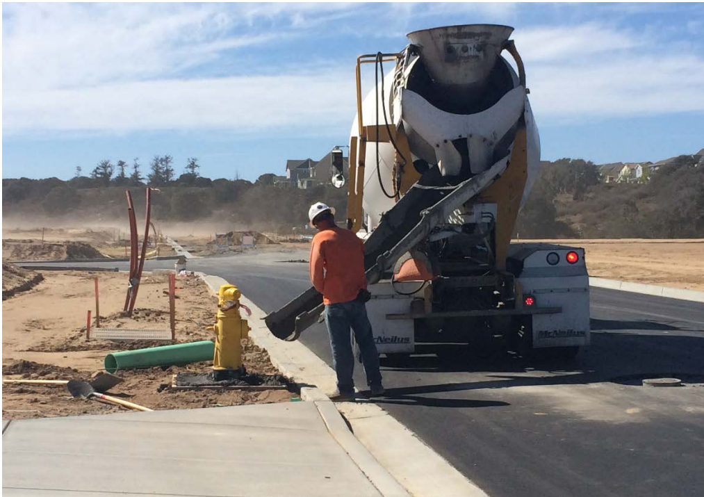
MCWD putting in water lines in East Garrison Phase 2, summer 2015.
