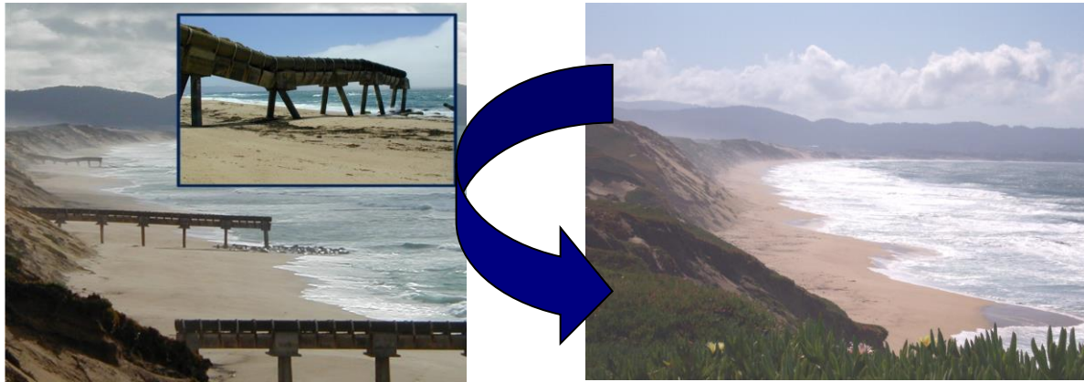
Storm drainage outfall removal – Before and After
